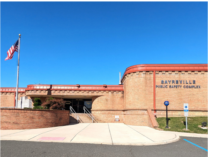
Sayreville Public Safety Complex
