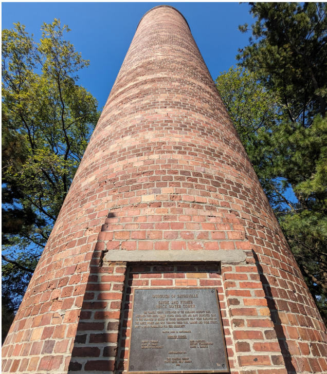
Sayre and Fisher Brick Water Tower
