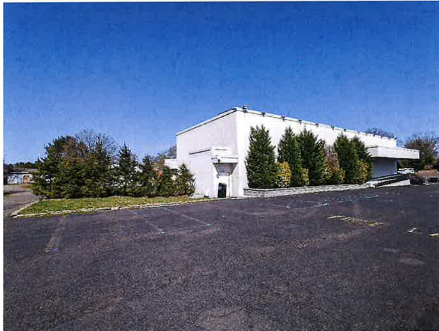
Figure 2 - Former Pure Nightclub Building
