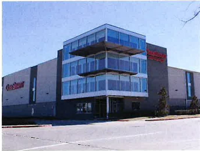
Figure 4 - Typical Modern Self-Storage Facility
