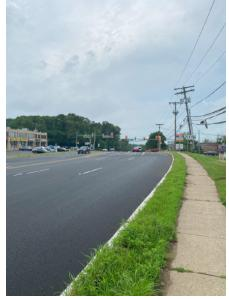
Westminster Boulevard: from Ernston Road to Meleta Way is a privately owned road oriented in the north/south direction with an approximate width of thirty (30') feet. The road has curb on both sides, and sidewalk on the western side for a majority of this stretch of road. The sidewalk has settled and is not ADA compliant. The roadway has numerous utility trenches, patches, and flat stretches that hold water. The entire road should be milled and repaved.
